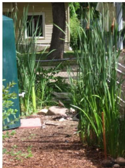
Rock and reed beds a few feet from the house provide filtering for grey water purification.
