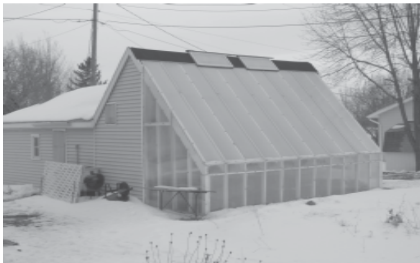
The surfaces with direct and maximum exposure to the sun are glazed with double-walled polycarbonate panels.
