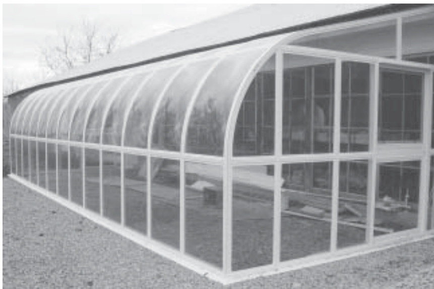
The greenbarn under construction at Windmill Point Farm.
